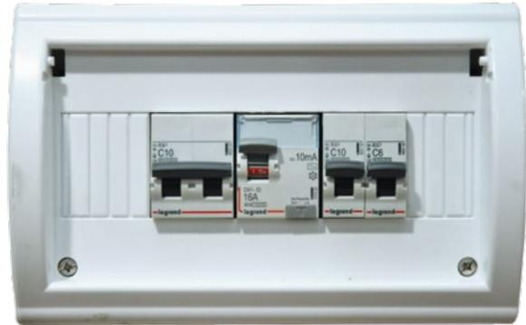
*The RCCB unit (centre) has an easily spotted test button marked 'T', which is a convenient indicator of the unit's operation status.*
